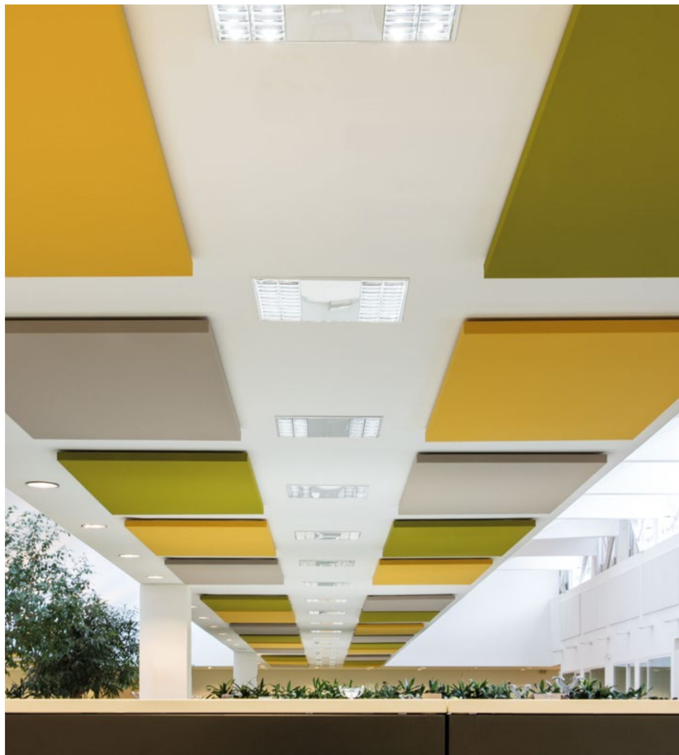
Siemens S.p.A. Milan, Italy
